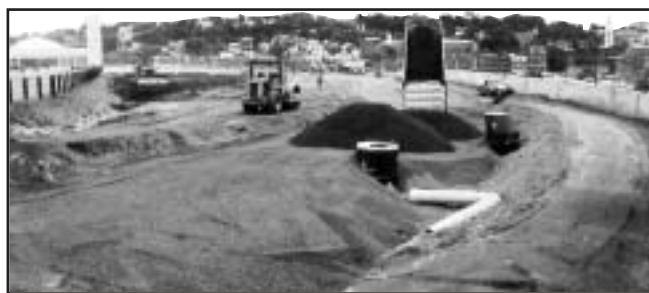
Retaining wall backfill, Providence, Rhode Island
