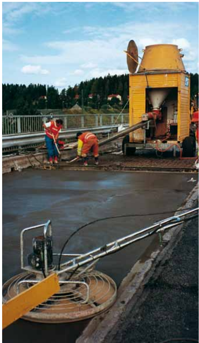
Bro under reparation
