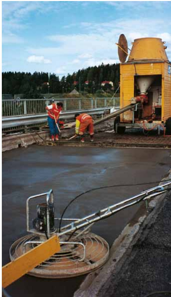
Bro under reparation
